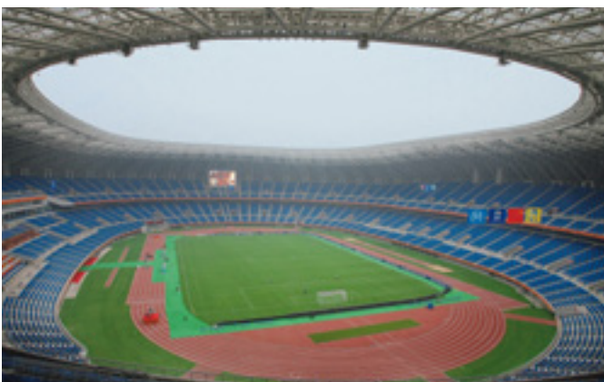
TIANJIN - Tianjin Olympic Center Stadium
