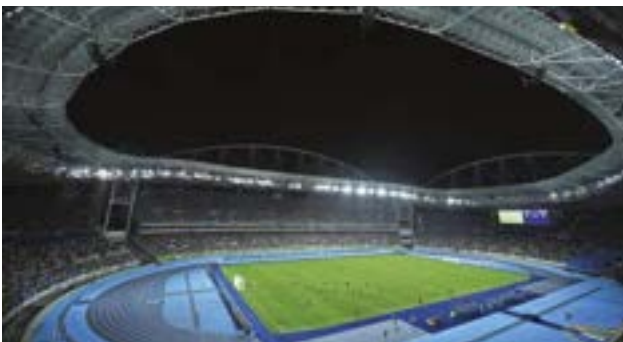
Rio de Janeiro, Olympic Stadium
